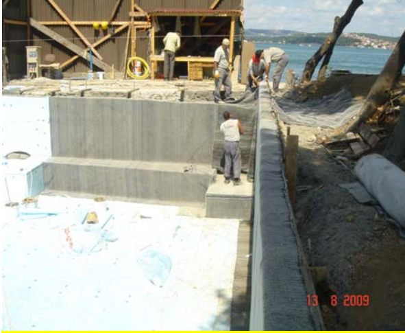
BentoShield roll should extend the wall at least 30cm.
