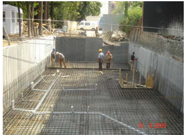
Reinforcing bars are directly placed on BentoShield MAX.
