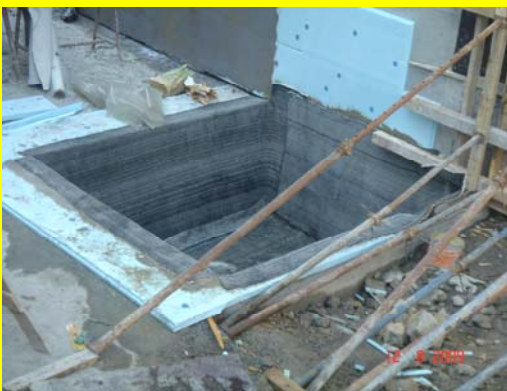
BS Granules sprinkled in overlaps of the elevator pit
