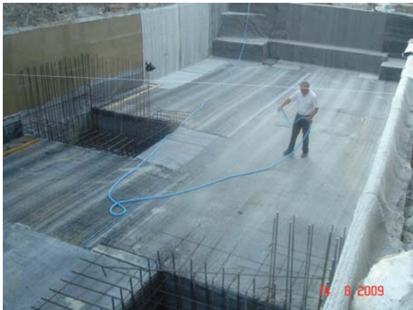
Before placing the bars and pouring the concrete, BentoShield is prehydrated.
