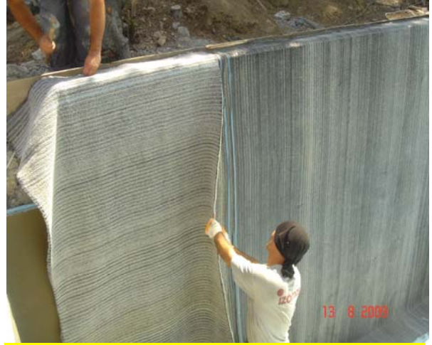
Two blue dashed lines assist the applicator for proper overlapping distance.
