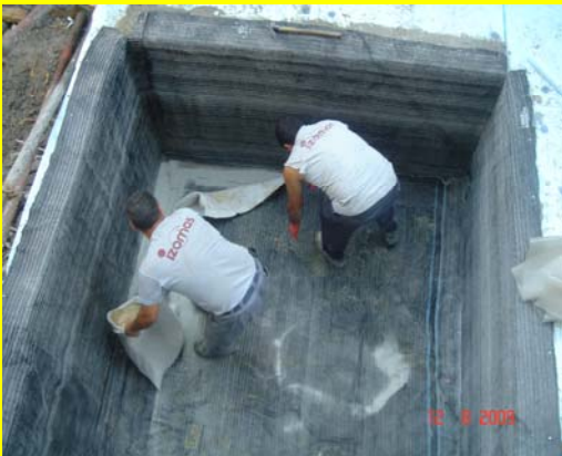
BS Granules sprinkled in overlaps of the elevator pit
