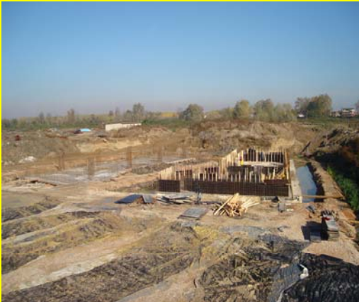
trenches around the foundation
